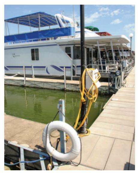
■ To help prevent the risk of electricity entering the water, have your boat and dock electrical systems checked regularly and make sure your electrical outlets have ground fault circuit interrupters (GFCIs).
