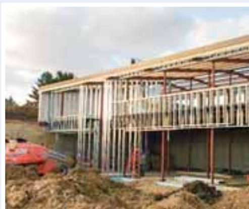
Work on the building addition at the Jo-Carroll Energy headquarters continues. Crews have been working on the geothermal wells, walls and roofing. Completion of the project is expected in July or August.
